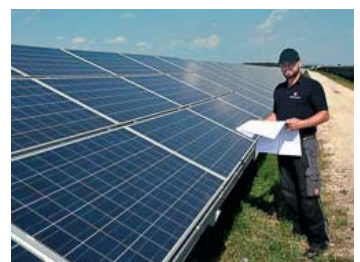
PI Berlin engineer inspects PV power plant
