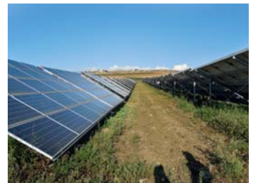
Examined PV power plant in Italy
