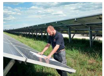
PI Berlin engineer inspects PV power plant
