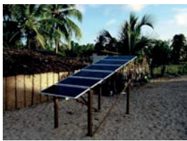
1b. Use of terrestrial PV has been for autonomous remote power supply (since 1980). System size has been in kW-ranges, PV system prices at 5\text{-}20 \text{ €/W}_p . PV electricity costs have been 1\text{-}2 \text{ €/kWh} and competed with battery power supply or diesel gen-sets.
