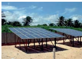
1b. Use of terrestrial PV has been for autonomous remote power supply (since 1980). System size has been in kW-ranges, PV system prices at 5\text{-}20 \text{ €/W}_p . PV electricity costs have been 1\text{-}2 \text{ €/kWh} and competed with battery power supply or diesel gen-sets.
