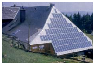
1b. Use of terrestrial PV has been for autonomous remote power supply (since 1980). System size has been in kW-ranges, PV system prices at 5\text{-}20 \text{ €/W}_p . PV electricity costs have been 1\text{-}2 \text{ €/kWh} and competed with battery power supply or diesel gen-sets.
