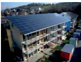
2. Due to grid-feed tariffs (FiT) in some countries, PV boomed during 2000-2010, production increased, prices went down. System size reached the MW-range and system prices at 2 \text{ to } 4 \text{ €/W}_p . PV electricity costs went down from 0.6 \text{ to } 0.2 \text{ €/kWh} .
